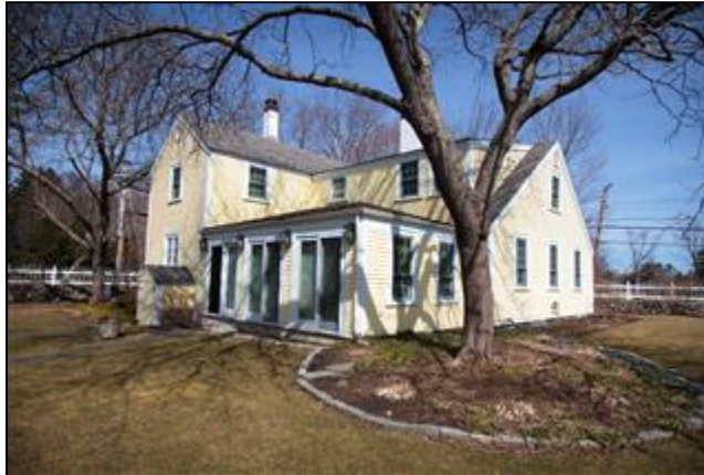
South East Corner
