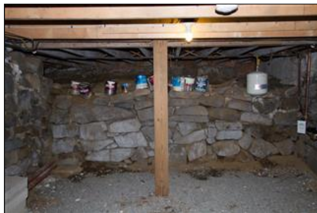
6.2 Picture 1 Wood Pier
