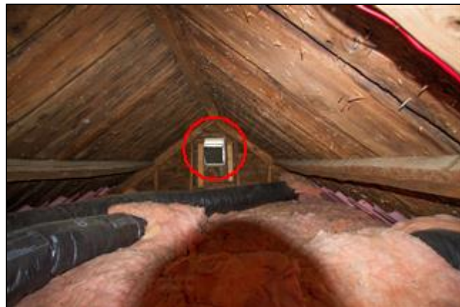
1.3 Picture 1 Gable vent
