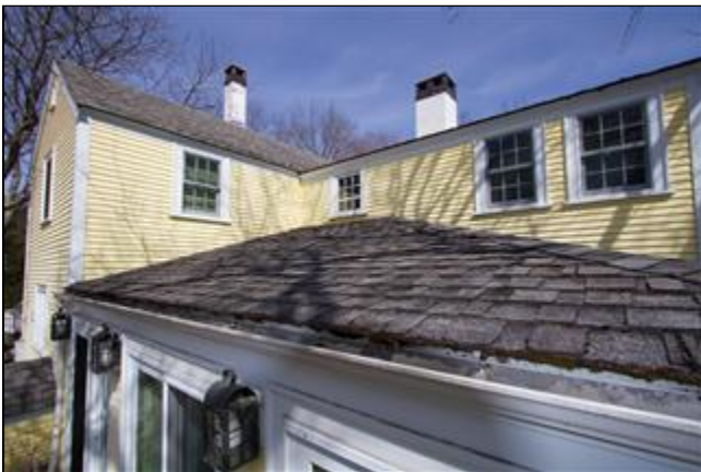
1.0 Picture 1 Sunroom Roof
