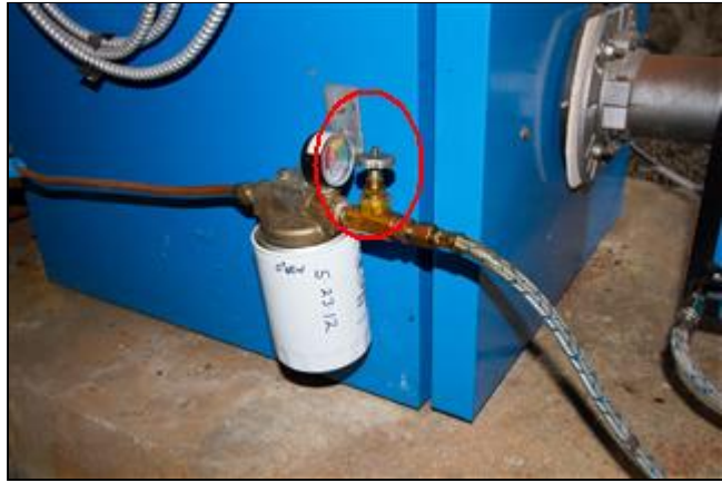
7.5 Picture 1 Fuel Shut Off
