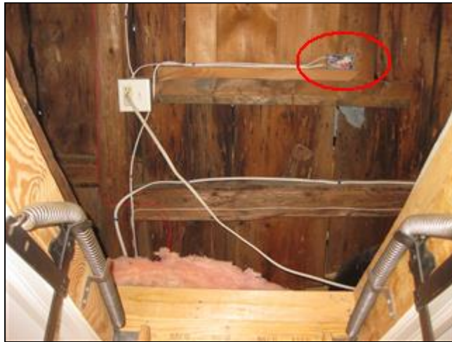
1.8 Picture 1 Cover Plate Needed
