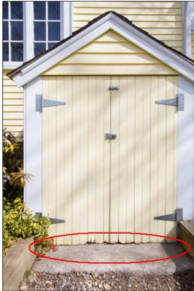
2.0 Picture 6 Basement Entrance
