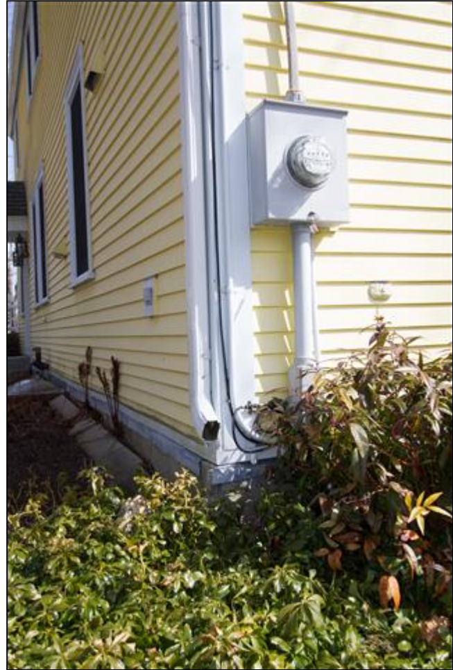
1.4 Picture 2 Downspout - South Corner
