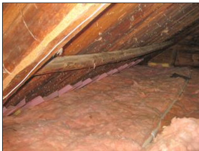
1.7 Picture 2 Attic Insulation
