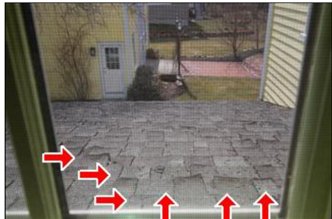
1.0 Picture 2 Sunroom Roof
