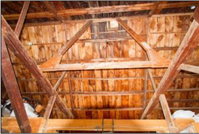
10.3 Picture 1 Roof Structure
