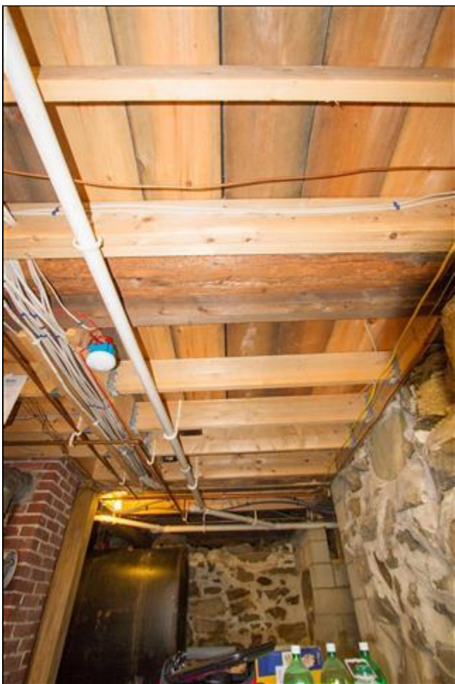
6.3 Picture 1 Floor below kitchen
