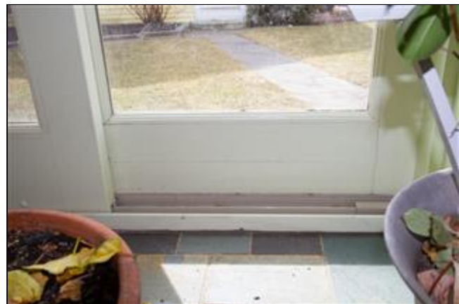
4.5.F Picture 2 Slider rail rot
