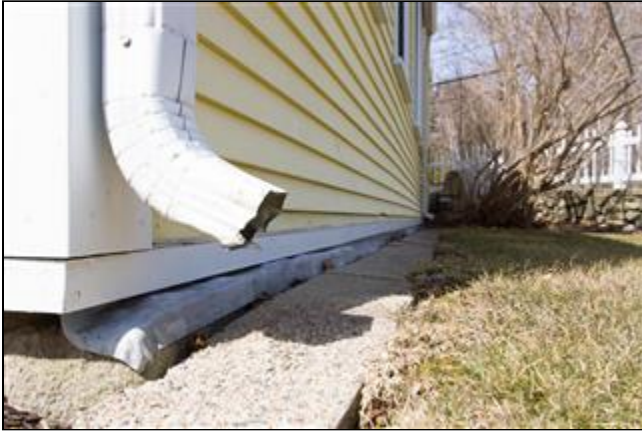
1.4 Picture 1 Downspout - North corner
