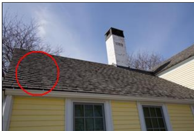
1.0 Picture 5 North Roof
