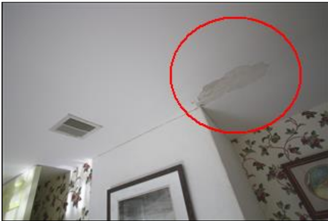
4.0.G Picture 1 Upstairs Bathroom
