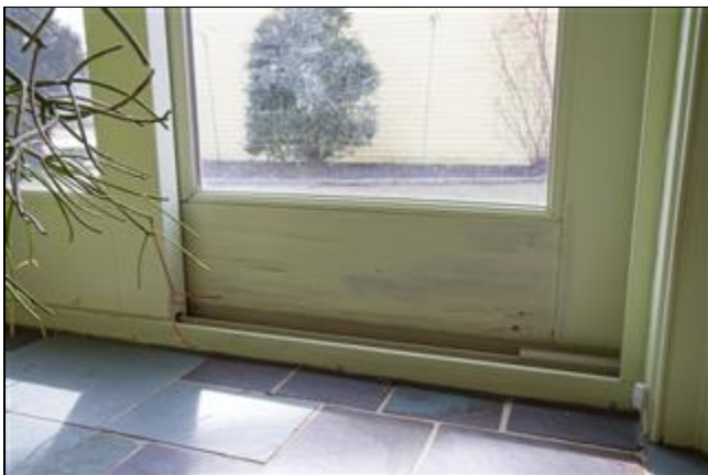
4.5.F Picture 1 Slider rail rot
