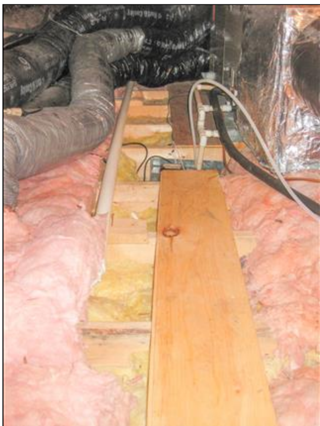
1.7 Picture 1 Attic Insulation
