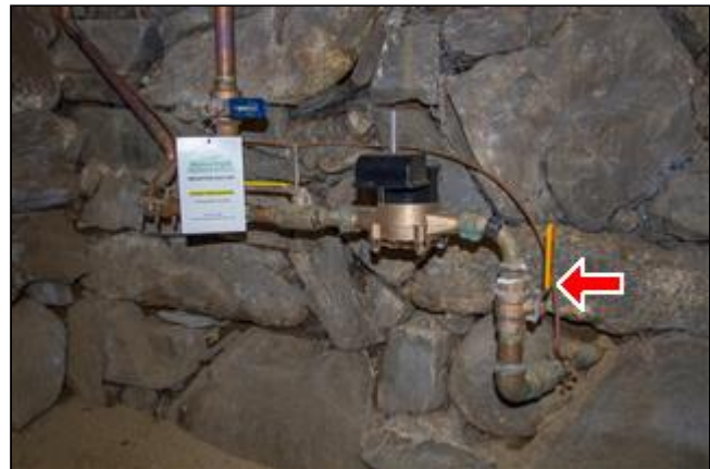
7.3 Picture 2 Interior Shut Off
