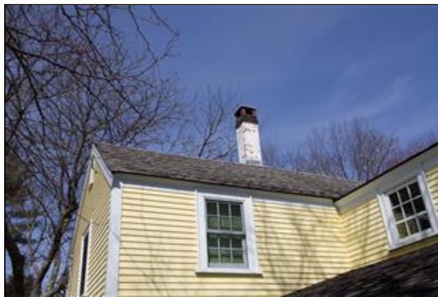
1.0 Picture 4 Upper Roof
