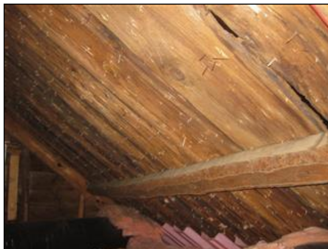
1.5 Picture 2 Roof Structure
