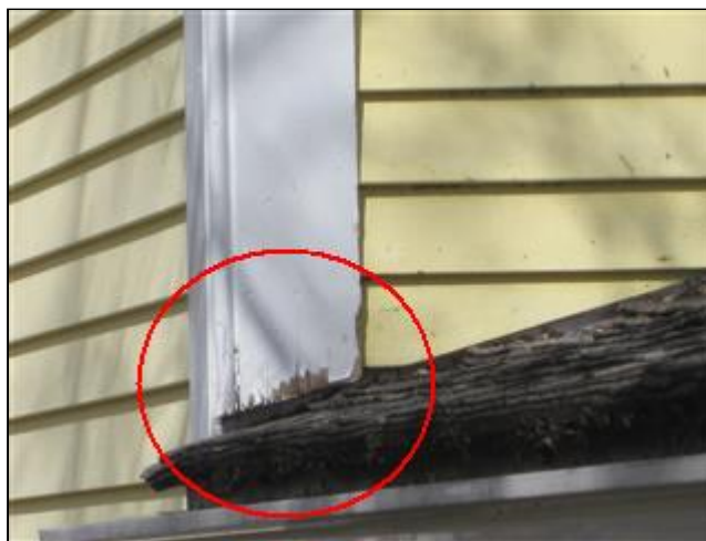
2.0 Picture 3 Corner Board
