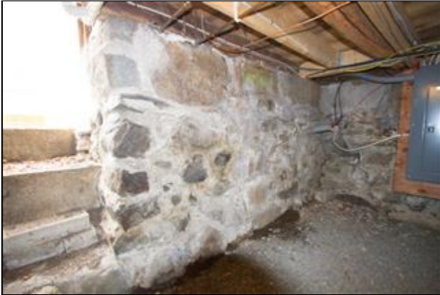
6.0 Picture 1 Stone Foundation
