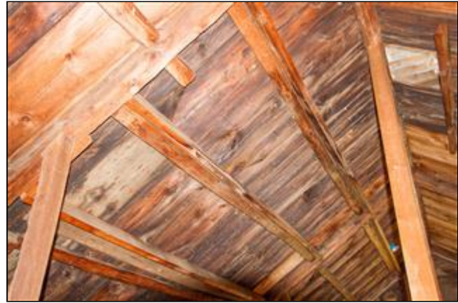
10.3 Picture 2 Roof Structure
