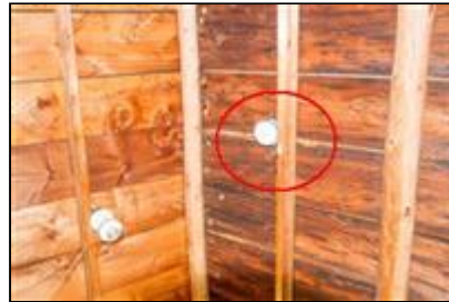
10.10 Picture 1 Smoke Detector
